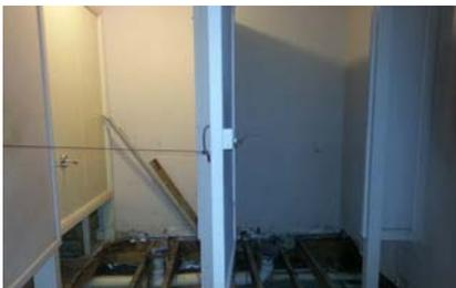
We had to remove the floor to fix a leak. This is only one of the problem areas in one of the bathrooms.
